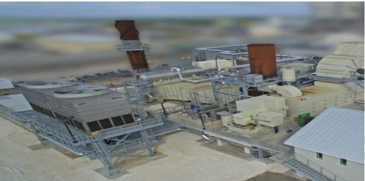
Eight Flags Combined Heat and Power Plant
