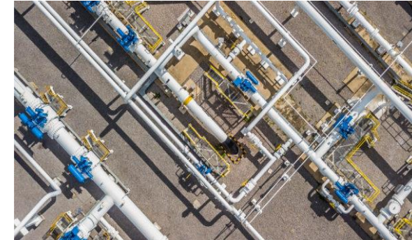
Pipeline Integrity Services
